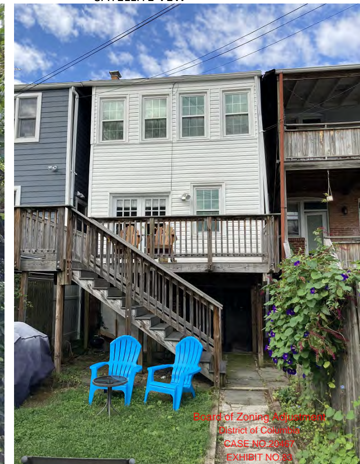
EXISTING REAR FACADE
