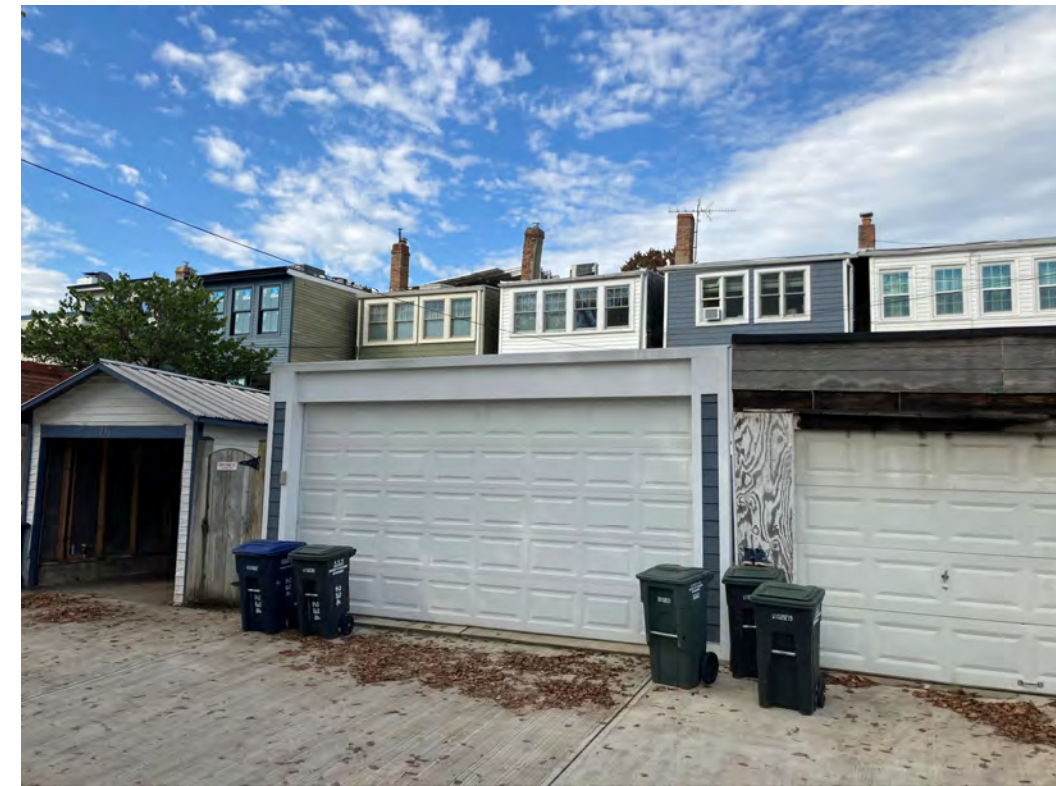
VIEW LOOKING SOUTH IN ALLEY
